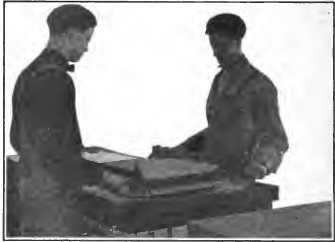
Stage 7—Dipping the other side of the section into the solder
